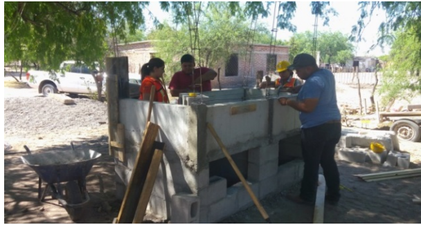
Figura 6. Muros base pets.
